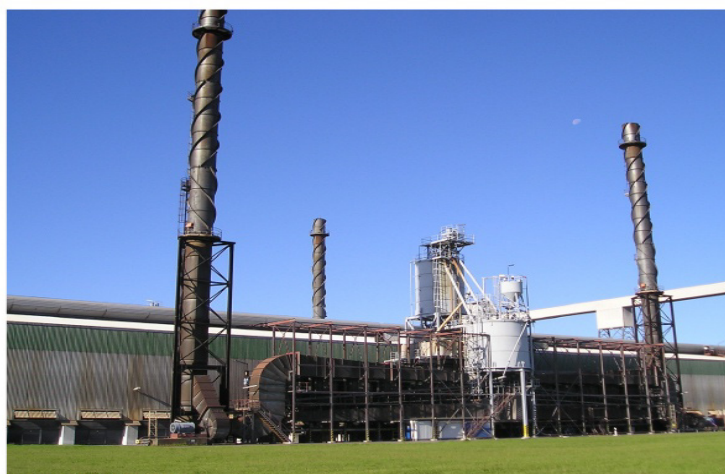
Figure 2. Gas treatment plant (SF3).
